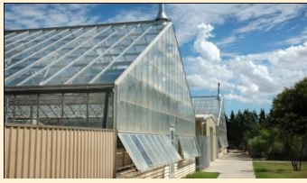
On-campus greenhouse and gardens facility
